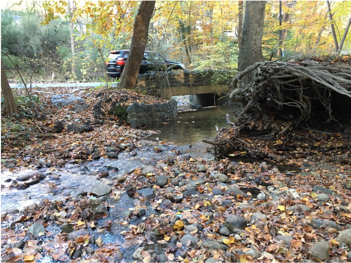
Figure 7: Normanstone Run monitoring site and bridge. Photo credit: Cathy Wiss.
