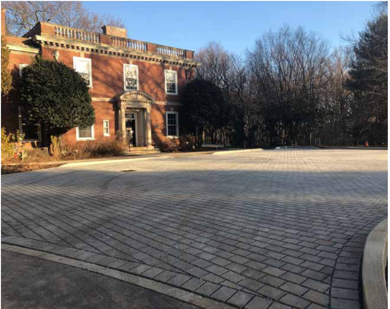
Permeable pavers treat and absorb stormwater outside ANS headquarters.
