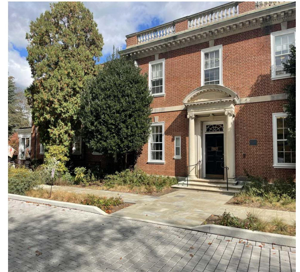
West Entry in fall; permeable pavers in foreground
