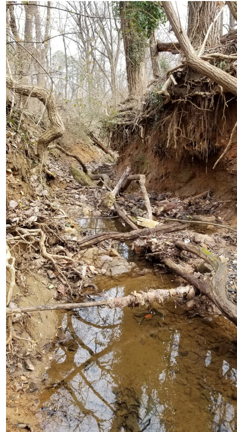
Severe erosion prior to restoration
