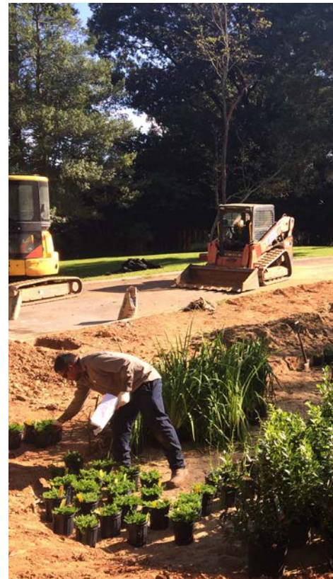
Rain Garden installation
