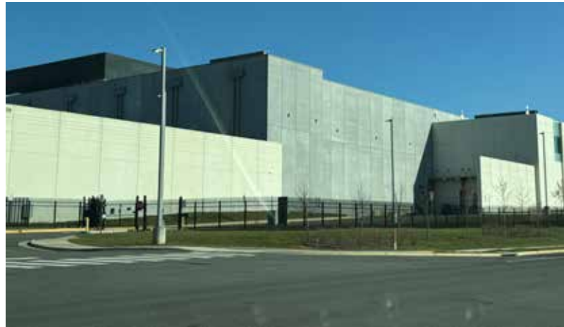
A data center in Loudoun County.
