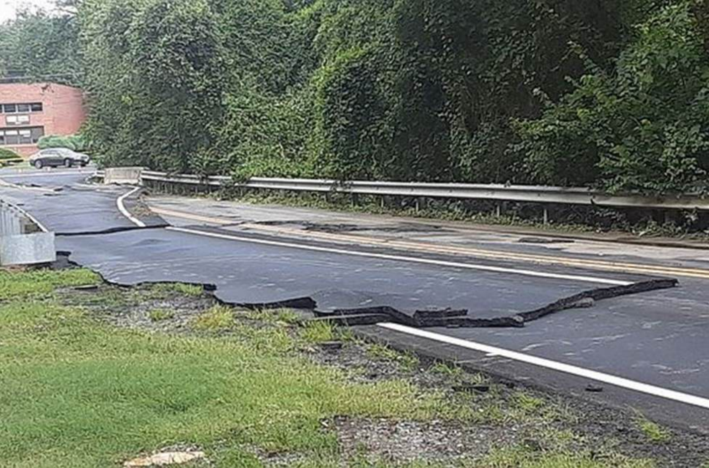
Newington Road damage, after flooding, near proposed trail entrance.
