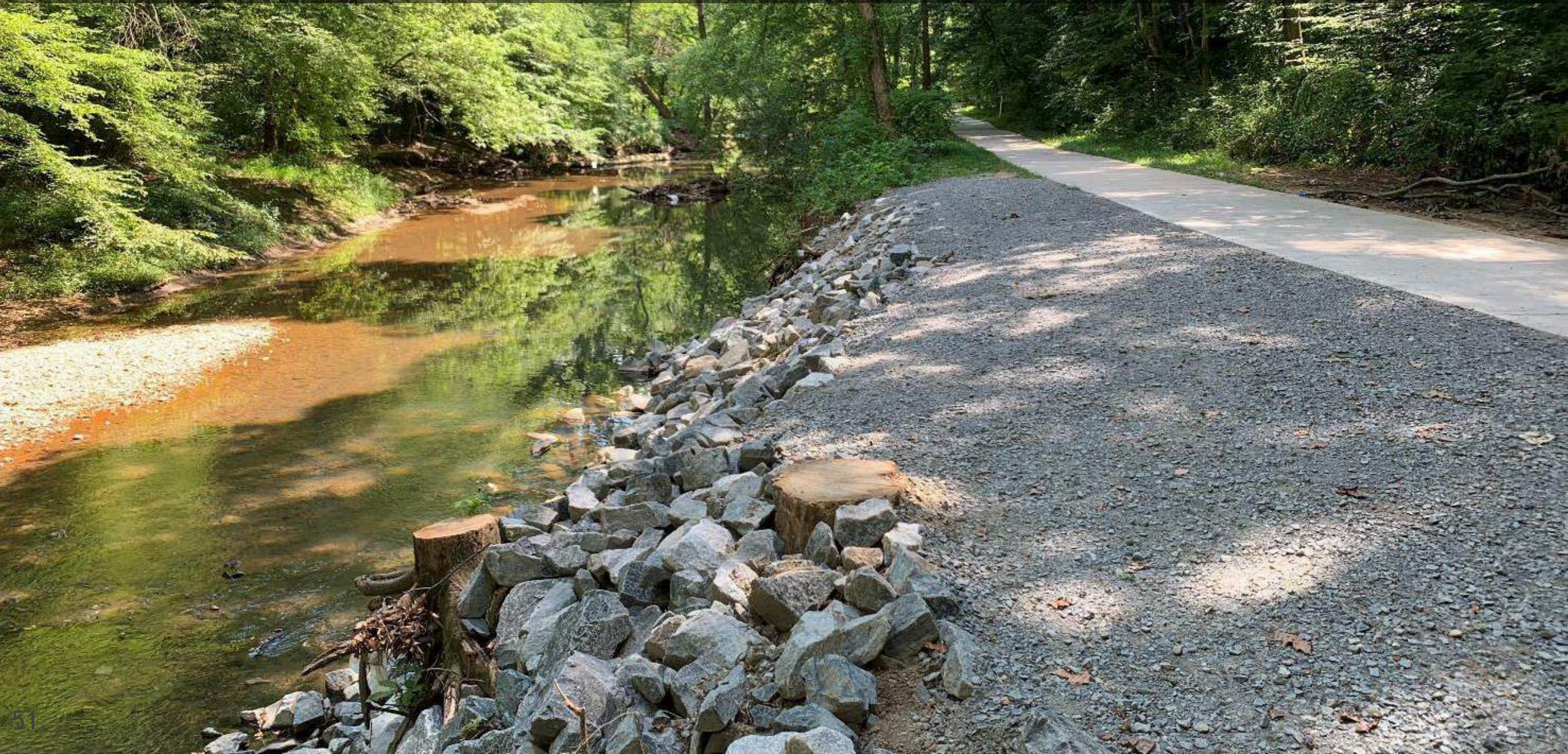
Cross County Trail, Fairfax County; reinforcement and hardening of riparian buffer. Photo courtesy of Friends of Accotink Creek
